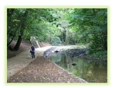
In 2021, NYCC completed a six week, £40,000 project to install stone gabions to rebuild the riverbank and resurface the footpath. This work has protected the Fairy Steps and will prevent future riverbank erosion in this area.
