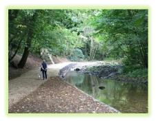
North Yorkshire County Council is responsible for maintaining public rights of way and accepted that this area of river bank needed to be repaired as a matter of urgency. Works were carried out in September 2021 and the riverbank has been fully reinforced with new gabions and the footpath refurbished with crushed stone.
